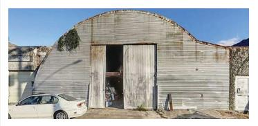
**The Moon at 631 Desire Street** is the renovation of an historic Quonset Hut structure located in New Orleans, Louisiana, USA. A Quonset Hut is a lightweight prefabricated structure of corrugated galvanized steel having a semicircular cross-section. Many were produced during World War II and military surplus was sold to the public. The development of the prototype is considered one of the first pre-engineered metal buildings.
